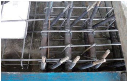
灌浆套筒及灌浆管安装
